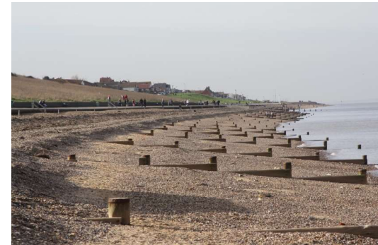
Promenade and Groynes at Minster (BA 11.1)
