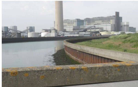
Kingsnorth Power Station (BA 1.2)
